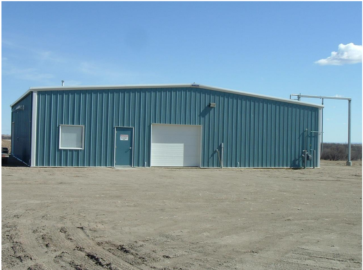
The Melita Water Treatment Plant
